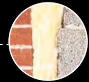
Increased Cavity Wall Thickness
