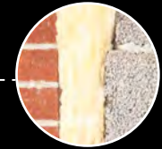
Increased Cavity Wall Thickness
