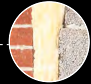
Increased Cavity Wall Thickness
